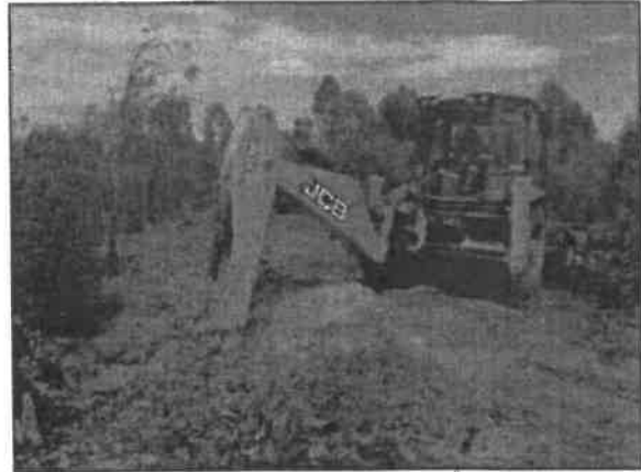
Plate 2: Site viewed towards the west at TP4
